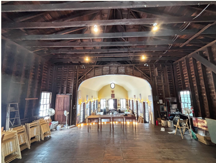
The stage and barrel-vaulted ceiling, looking south toward the assembly room.
